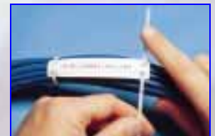
Attach marker to cable with Panduit cable ties
