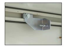
B) Secure the bottom panel supports and the upper panel mounting brackets into place. To make sure the inner panel is straight, line up the back face of the upper mounts to the back face of the bottom supports. Use the notches in the frame for guidance.
